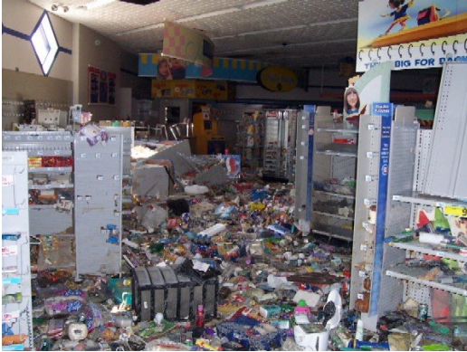
Hurricane Damage - Interior
